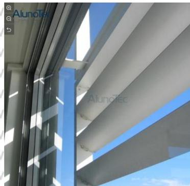
Gambar 4 29 Aluminium Aerofoin Sun Louvres
