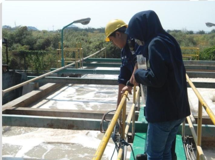
Gambar 14. Pengambilan Sampel Aeration Tank
