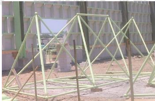
Gambar 2.11 Pipa Space Frame
