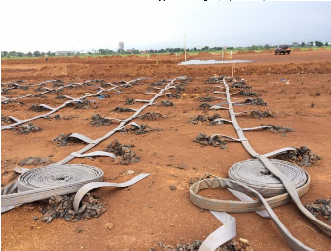
Gambar 2.1.33 PHD metoda Preloading
