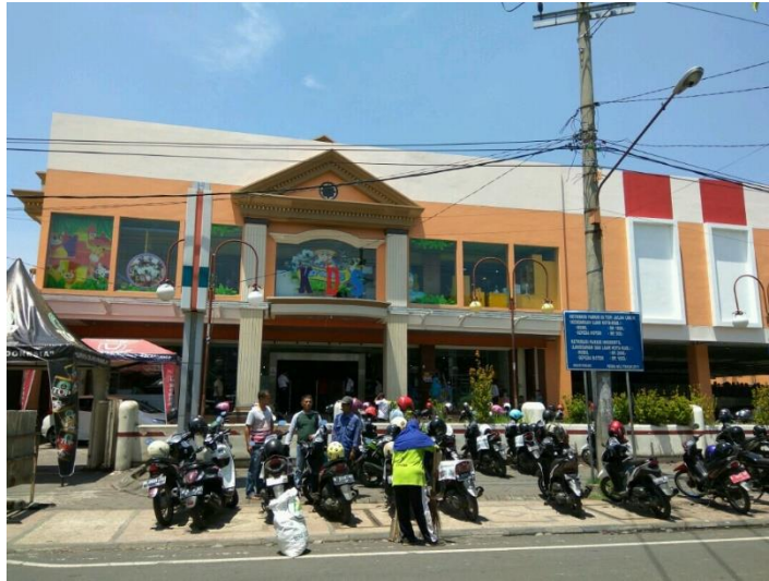
Tampak Depan Supermarket KDS
