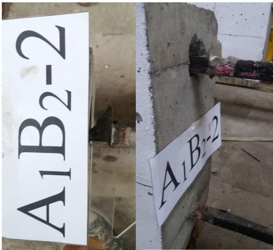
Gambar Keruntuhan Benda Uji Pull Out A 1 B 2 – 2
