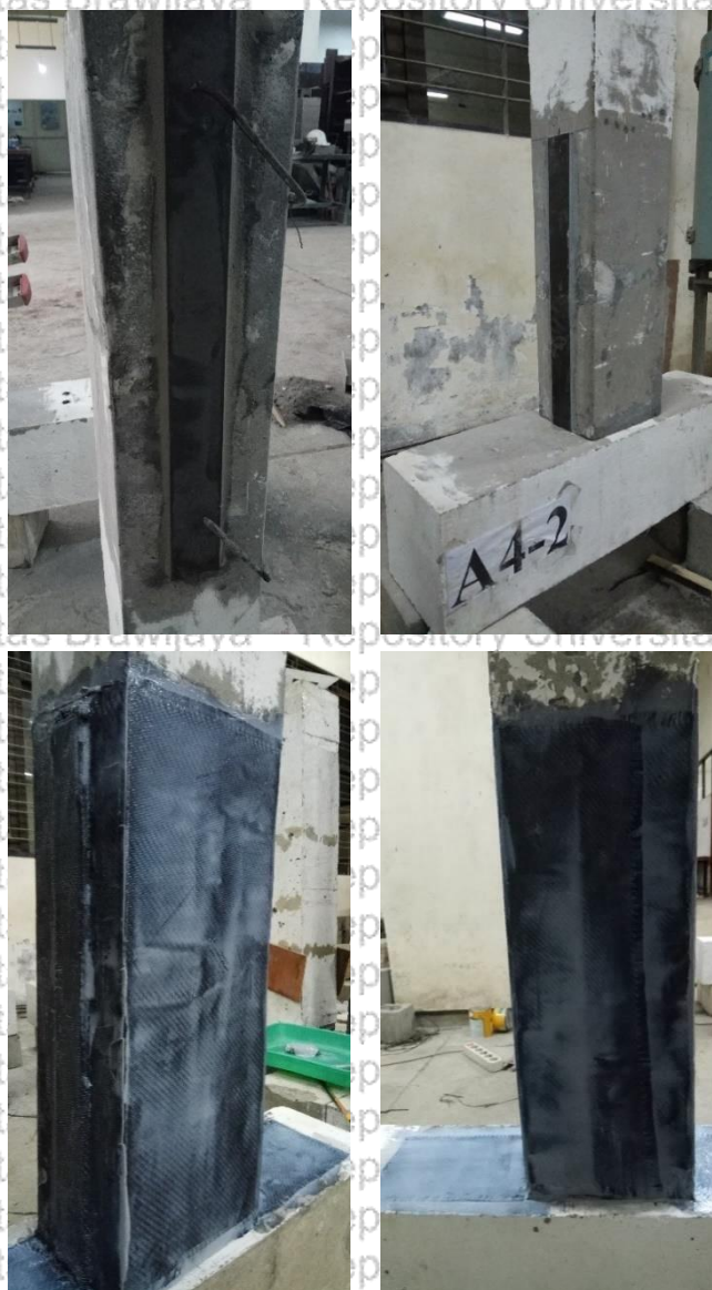
Gambar 5.8 Benda uji retrofitting
