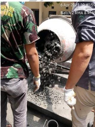
Gambar 2. Proses *Mixing* Material
