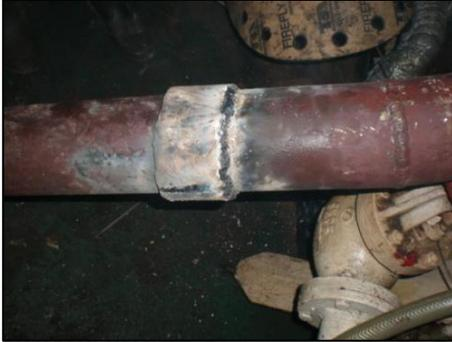
Gambar 2.7 Galvanic corrosion
