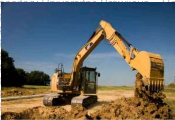
Gambar 2.6 Excavator Sistem Hidraulik Sumber : Caterpillar (2012)
