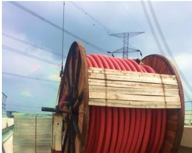
Gambar 4.2 Power cable 20 KV
