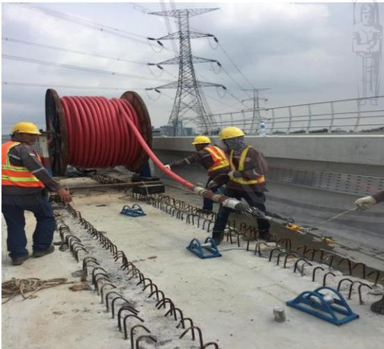
Gambar 4.15 Pulling Cable Internal
