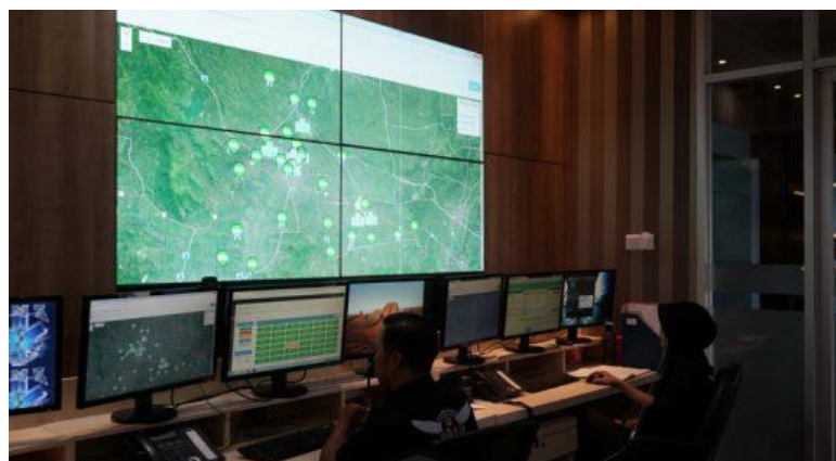
Ruang Public Safety Center (PSC)
