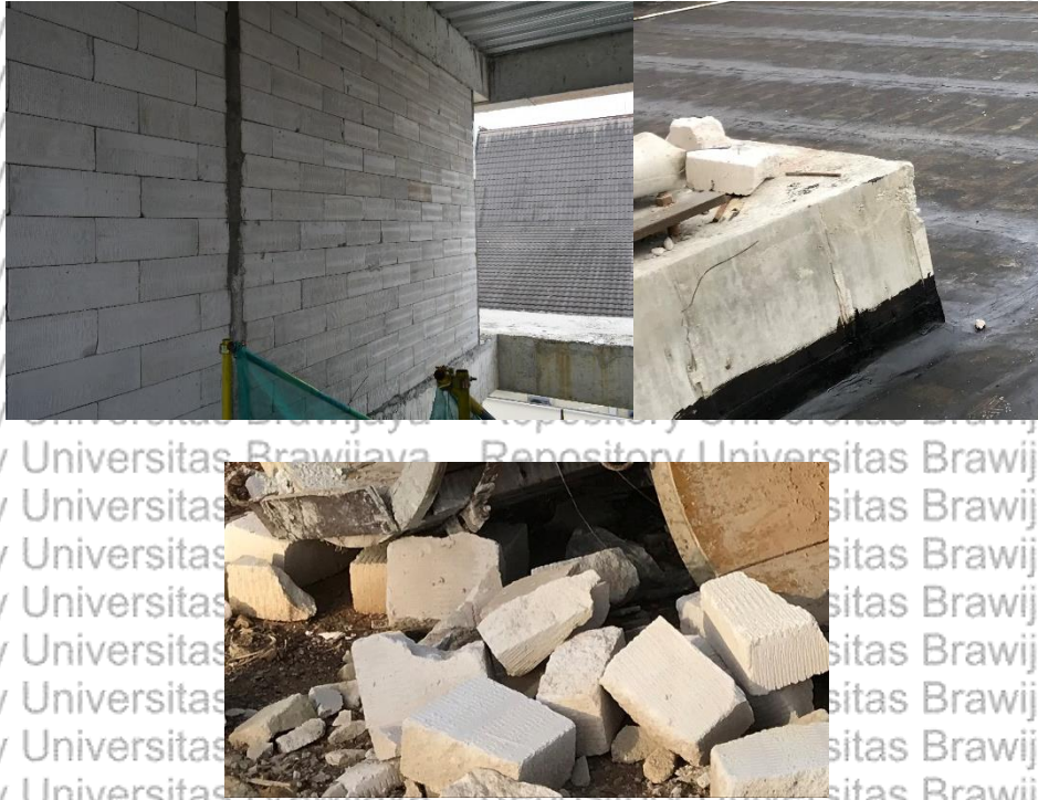
Gambar 4.134 Sisa Material Bata Ringan
