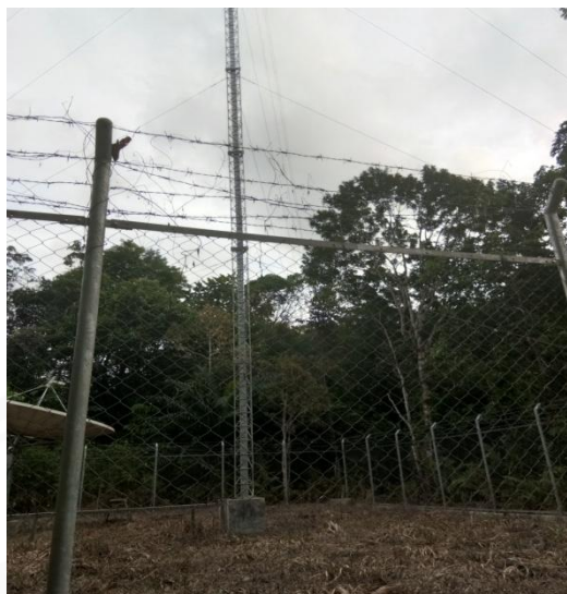
Gambar 4.8 Bangunan BTS ( Base Transceiver Station ) di Desa Lauk
