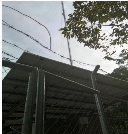
Gambar 4.9 Bangunan BTS ( Base Transceiver Station ) Desa Sungai Uluk Palin
