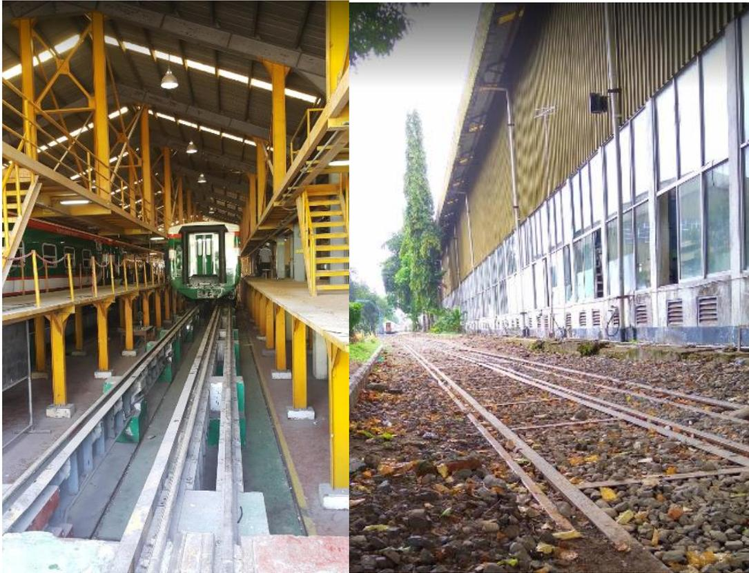
**Gambar 4. 26.** Tampak Bangunan *High Bay and Monitor Types*
