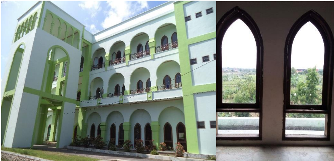
Gambar 3.2 Gedung Islamic Center Pamekasan
