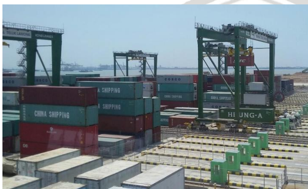
Gambar 4.9 Automated stacking crane Sumber: PT. Terminal Teluk Lamong (2017)
