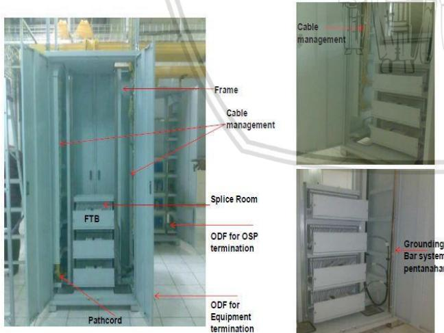
Gambar 2.15 Optical Distribution Frame (ODF)
