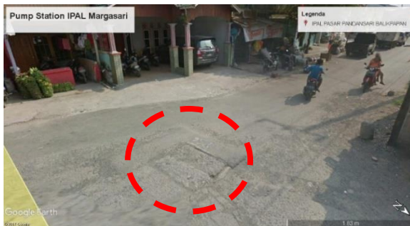
Gambar 4.9. Pump Station IPAL Margasari Kecamatan Balikpapan Barat Sumber : Google Earth, 2017
