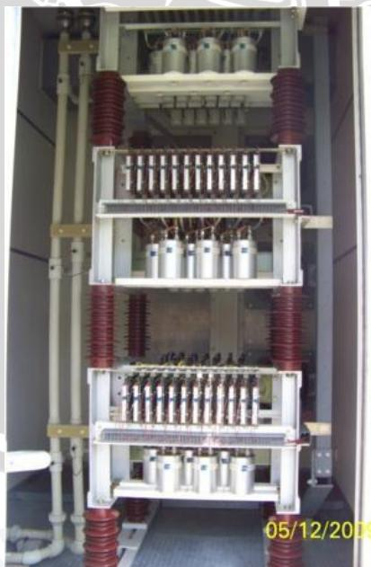
Gambar 2. 11 Thyristor valve tower
