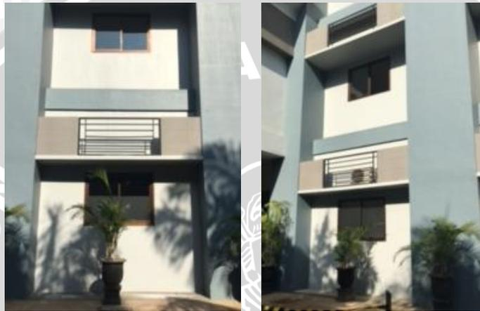
Gambar 4. 20 Foto shading device eksisting
