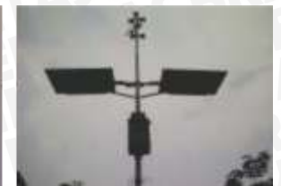
CCTV/Remote Monitoring System Tenaga Surya
