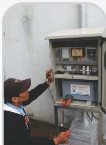
SOLAR BATTERY TEST
