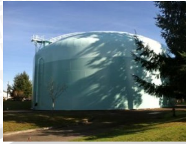
Gambar 2.16. Water Tank Sumber : http://www.oakharbor.org
