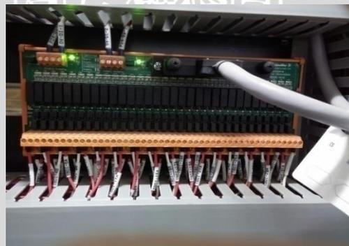
**Gambar 3. 14 Port *Output* Digital DCS**
