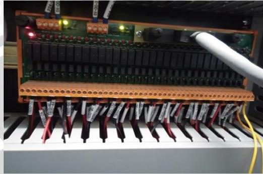
**Gambar 3. 13 Port *Input* Digital DCS**
