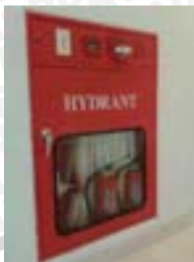
Gambar 4. 81 Hydrant Box Sumber: cv_kartika_sari_indonetwork.co.id
