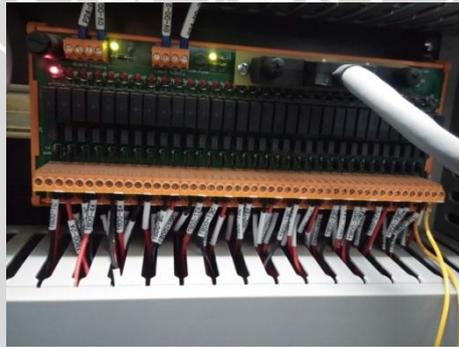
Gambar 3. 6Port Input Digital DCS
