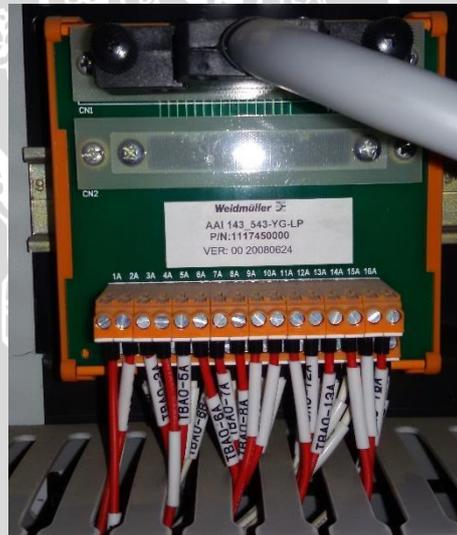
Gambar 3. 8Port Input Analog DCS
