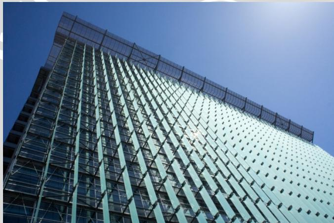
Gambar 2.20 *Shading device* vertikal.
