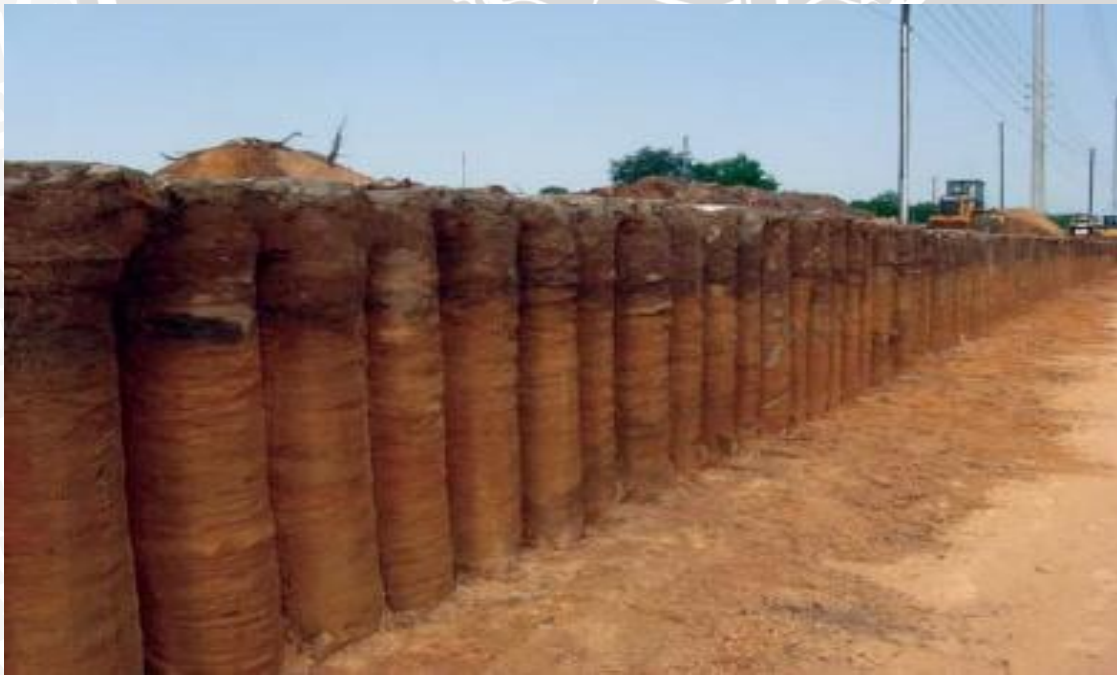
Gambar 2.5 Kolom stabilisasi hasil deep soil mixing
