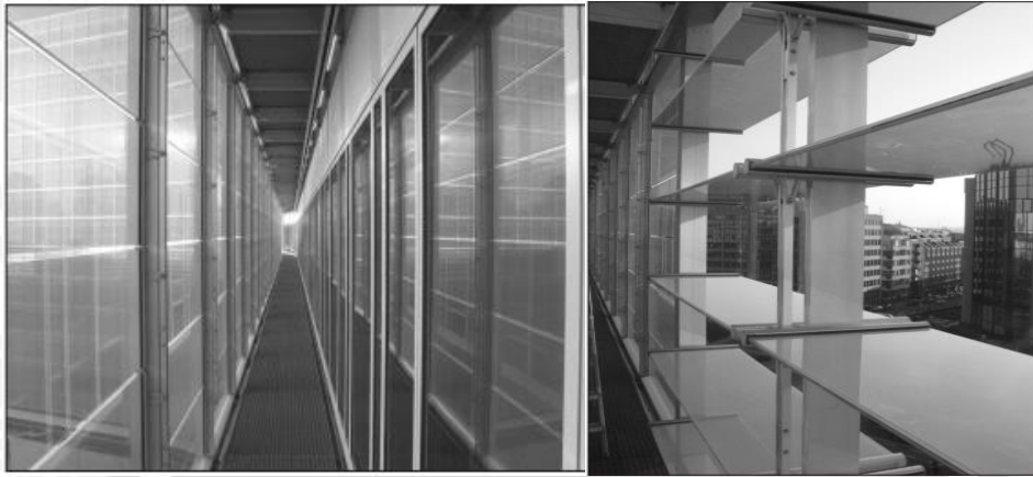
gambar 2.13 Multi Storey Louver (sumber : www.cstc.be )
