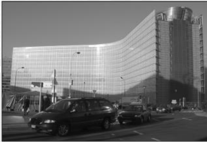
gambar 2.12 Berlaymont Building (sumber : www.archdaily.com )
