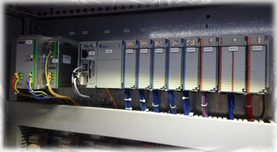
Gambar 2.3 PLC CompactLogix 1769-L32E OK Mill
