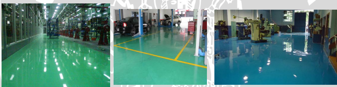
Gambar 4. 59 Lantai Epoxy
