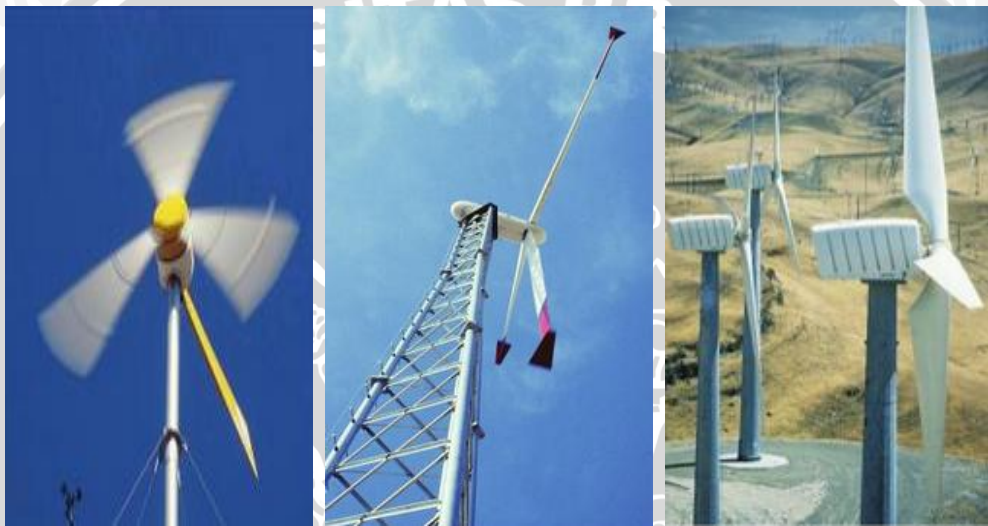
Gambar 2.5 Turbin angin horizontal.
