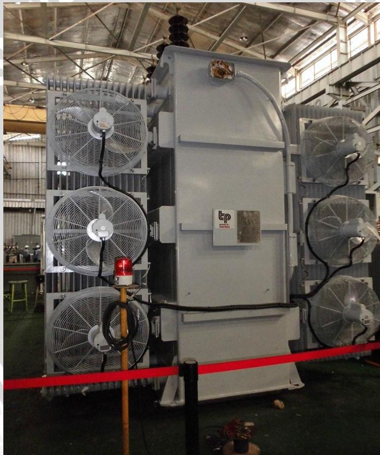
**Gambar 4.1** Transformator Distribusi 20 MVA
