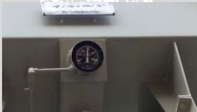
Gambar 4. 2 Oil Level Indicator Sumber : PLTA Sutami
