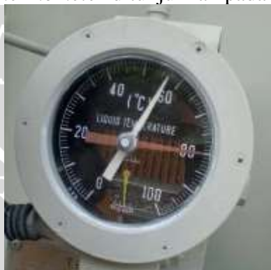
Gambar 4.5 Oil Thermometer Sumber : PLTA Sutami
