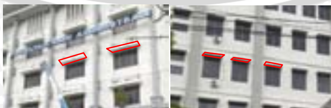
Gambar 4.18 Penerapan overhang
