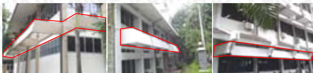
Gambar 4.14 Penerapan panel/awning
