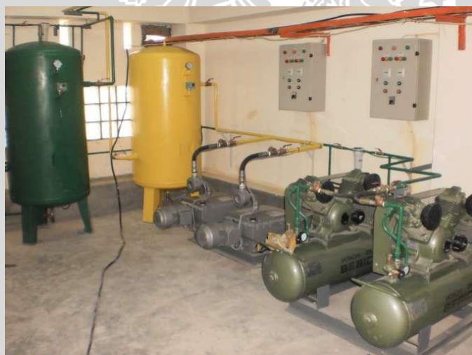
Gambar 4.16 Gas medis sentral (Sumber: www.google.com/gas_medis )
