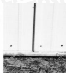
Fig. 12. Metal siding may provide entry points for mice and rats where panel ends are left open (left). Properly installed metal siding rests on the concrete floor or has metal flashing or angle iron to block entry (right).
