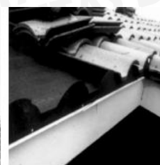
Fig. 25. "Bird stop" shaped metal for tile roofs to prevent rodent and bird entry. (Fig. 23).
