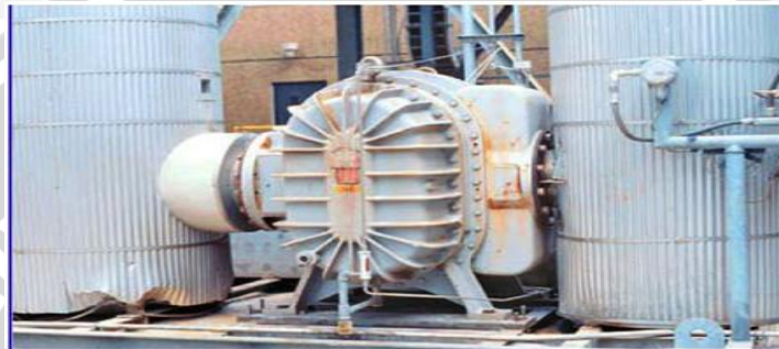
Figure 1 - Roots-type positive displacement blower at a petrochemical plant. (Source: Lubrication Systems Company, Houston, Texas)
