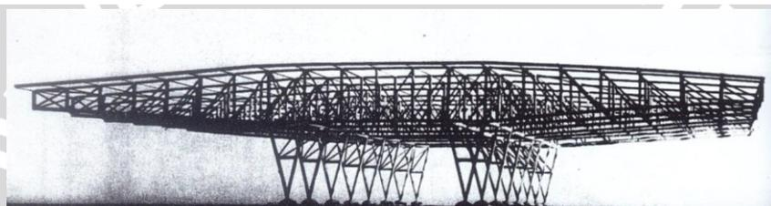
Gambar 2.29 System of flat trusses with large cantilevers at both ends
