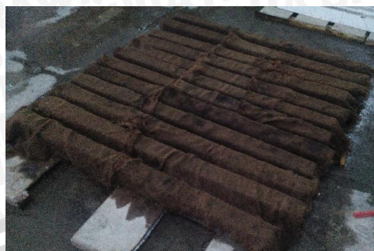
Proses Curing Balok
