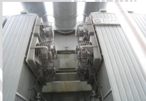
Gambar 2.8 Kipas Pendingin Transformator
