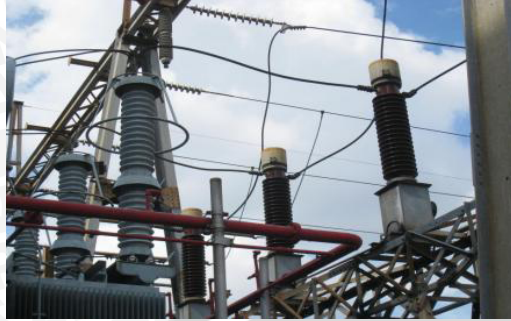
Gambar 2.5 Bushing Transformator
