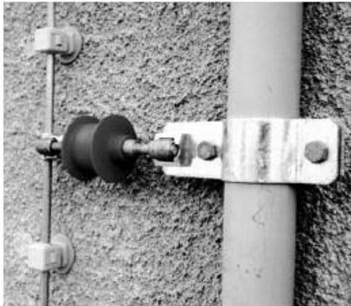
*Figure 5.7 b Isolatng spark gap for isolatng metal systems of different potentials*
