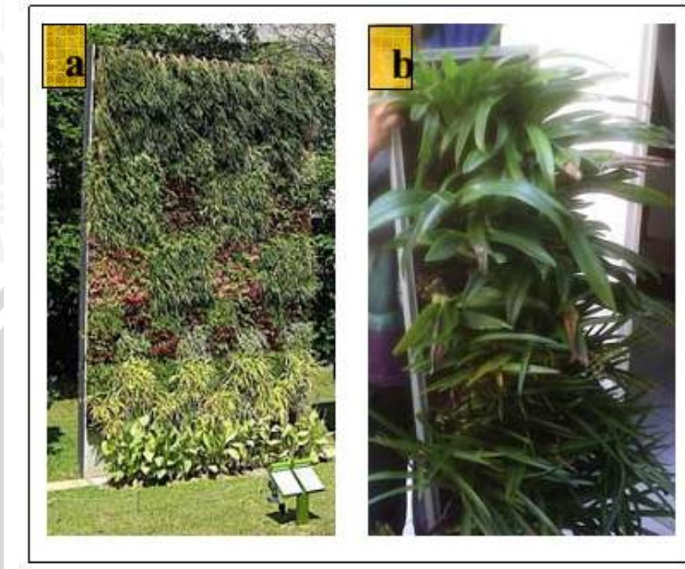
Gambar 2.15 Carrier type (a. Planter pocket, b. Porous)
