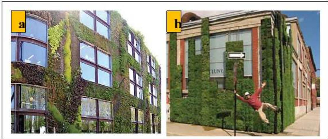
Gambar 2.18 *Structure subclass (a. Individual mounting, b. Group mounting)*
