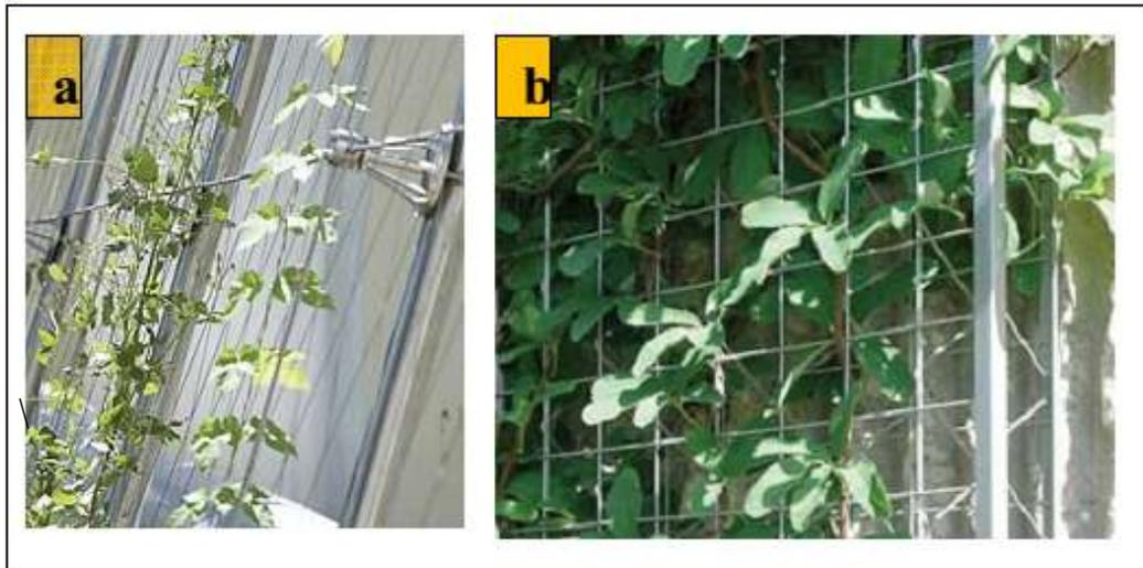
Gambar 2.16 Support type (a. Singular, b. Mesh)
