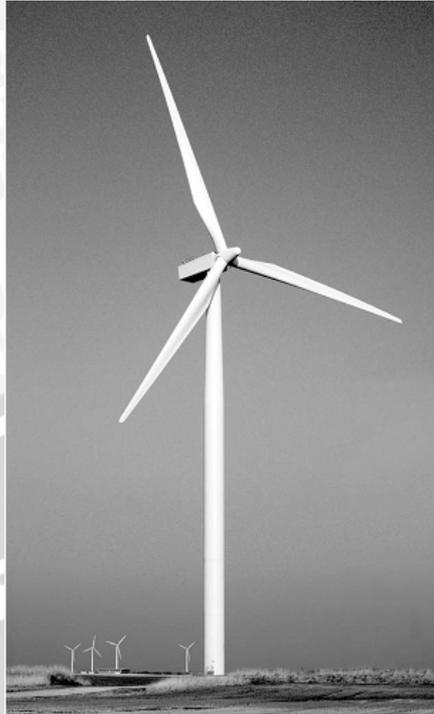
Gambar 2.2 Turbin Angin Sumbu Horizontal
