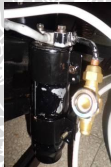
Gambar 3.6 Filter drier
