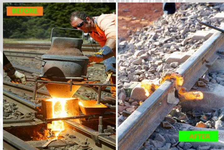
Gambar 2.8 *Thermit Welding*
