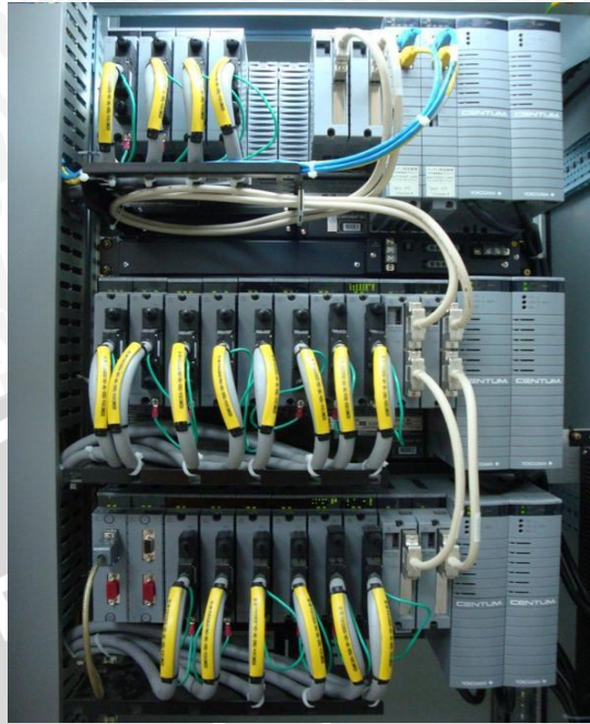
Gambar 2.9 Distributed Control System
