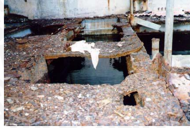
Gambar 2.1 Uniform Corrosion Sumber : NASA, Corrosion Division
