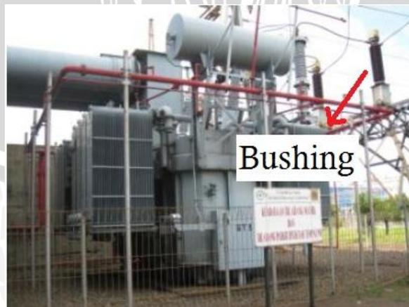
Gambar 2.5 Bushing Transformator
