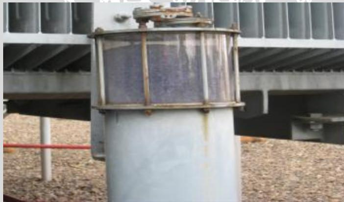
Gambar 2.10 Alat Pernafasan Transformator
