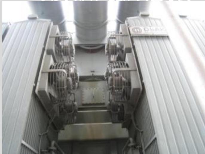
Gambar 2.8 Kipas Pendingin Transformator
