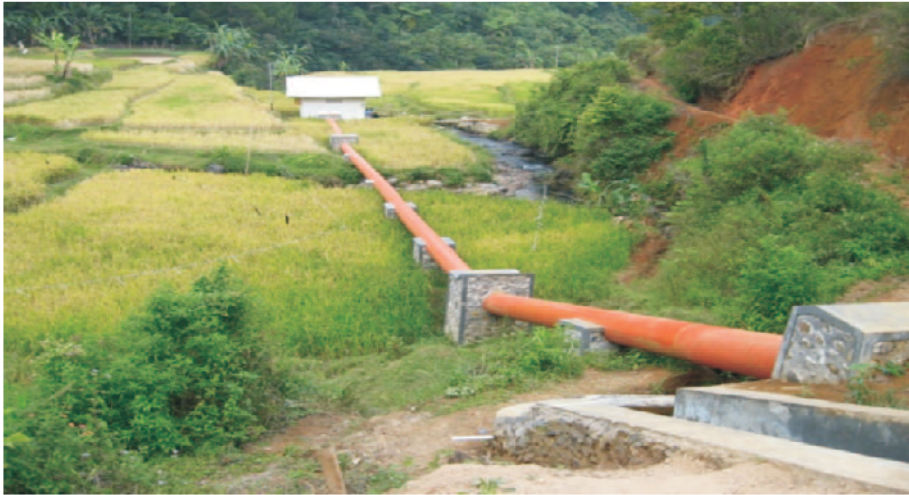
Gambar 2.16 Pipa Pesat ( Penstock )
